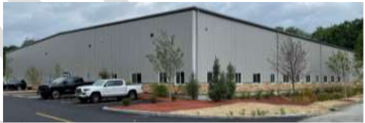
Accumet Engineering new building shell at 41 Lake George Street – July 2023
