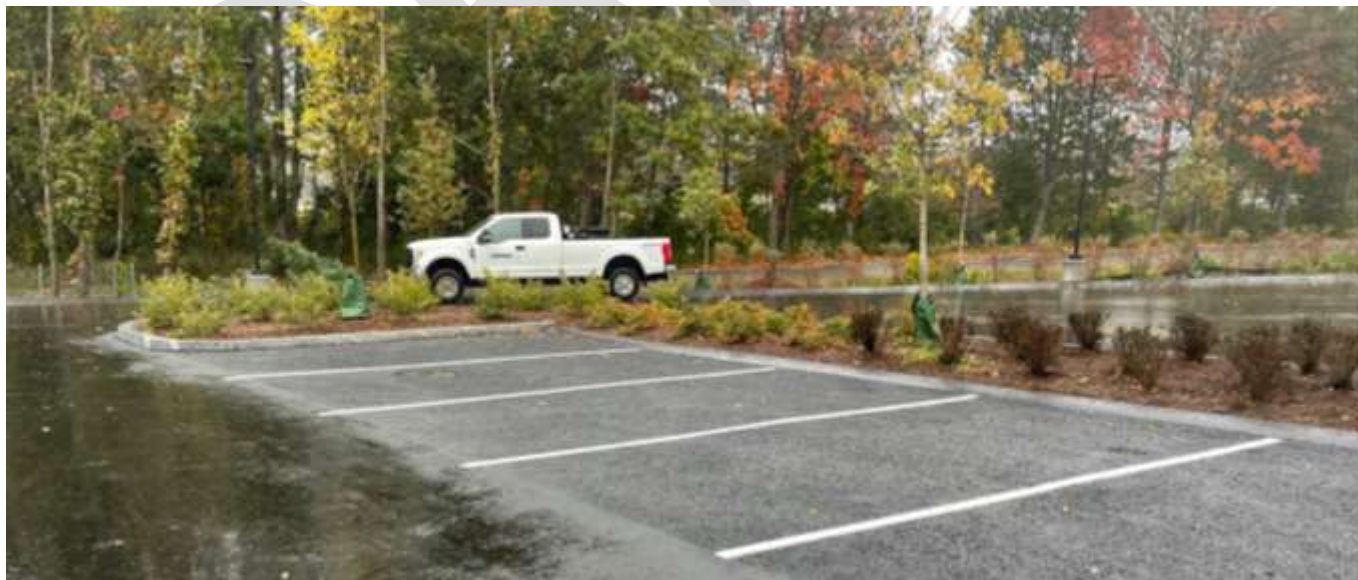
Existing Porous pavement parking spaces and bio-filtration landscape islands behind 33 Jackson Road. – September 2023
