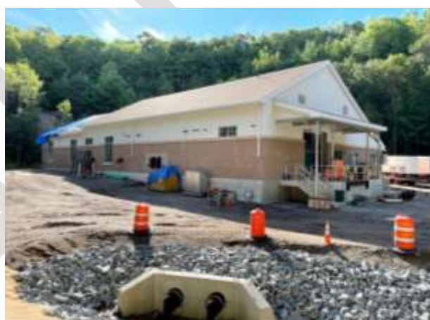
New Shabokin Water Treatment Facility off Sheridan Road: August 2023
