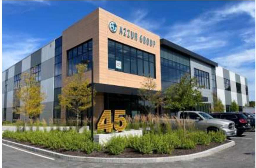
Front view of 45 Jackson Road - July 2023
