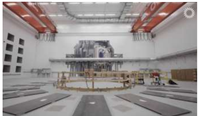
*Interior of SPARC – (“Tokamak Hall”) under construction – August 2023
